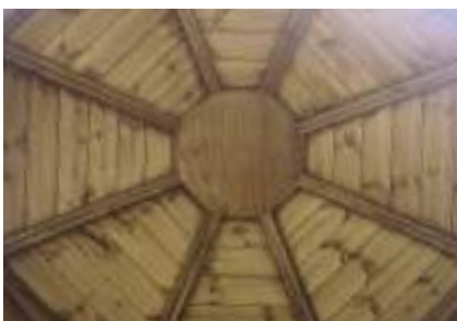
Internal roof structure
