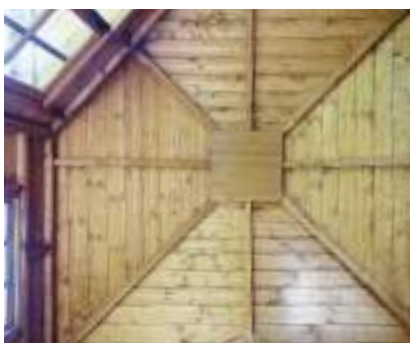
Internal roof structure
